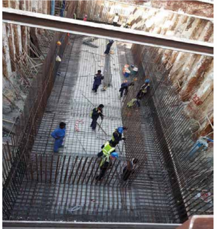
Steel Reinforcement Works for HB Office Space Construction at Yas Island, Abudhabi U.A.E.
